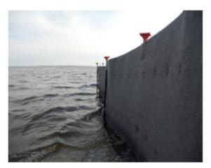
Silt fence is made of a woven polypropylene material and it is n o n - b i o d e g r a d a b l e . T h i s engineered geotextile is stabilized to resist degradation due to ultraviolet exposure. It is resistant to commonly encountered soil chemicals, mildew and insects.
