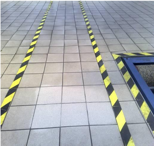
The results when used on a workshop tiled floor
